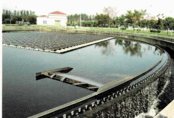
Sewage treatment reservoir
