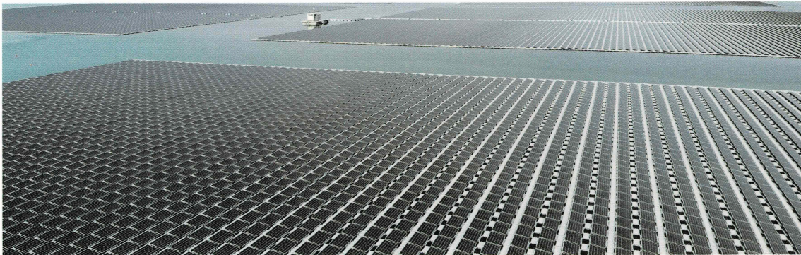
Guqiao Huainan • China Installed capacity : 150MW
